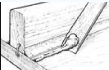
Figure 14 Clean up the excess epoxy outside the fillet margin.
